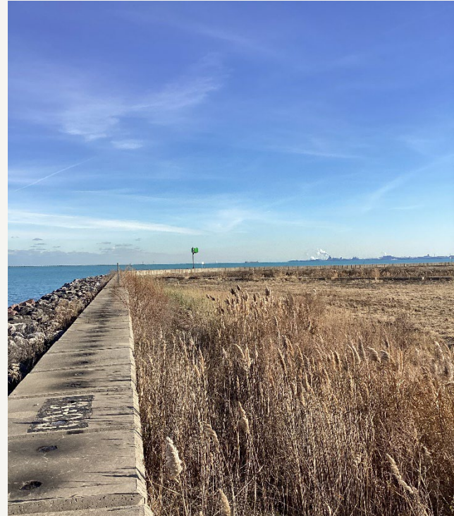
Army Corp's Calumet Harbor and River Confined Disposal Facility (CDF)
